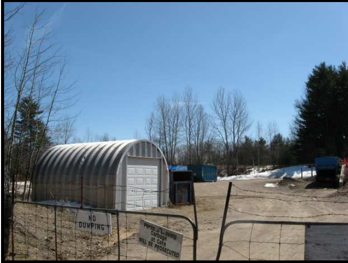
Photo 1. Ruby Road waste site viewed from entrance gate
